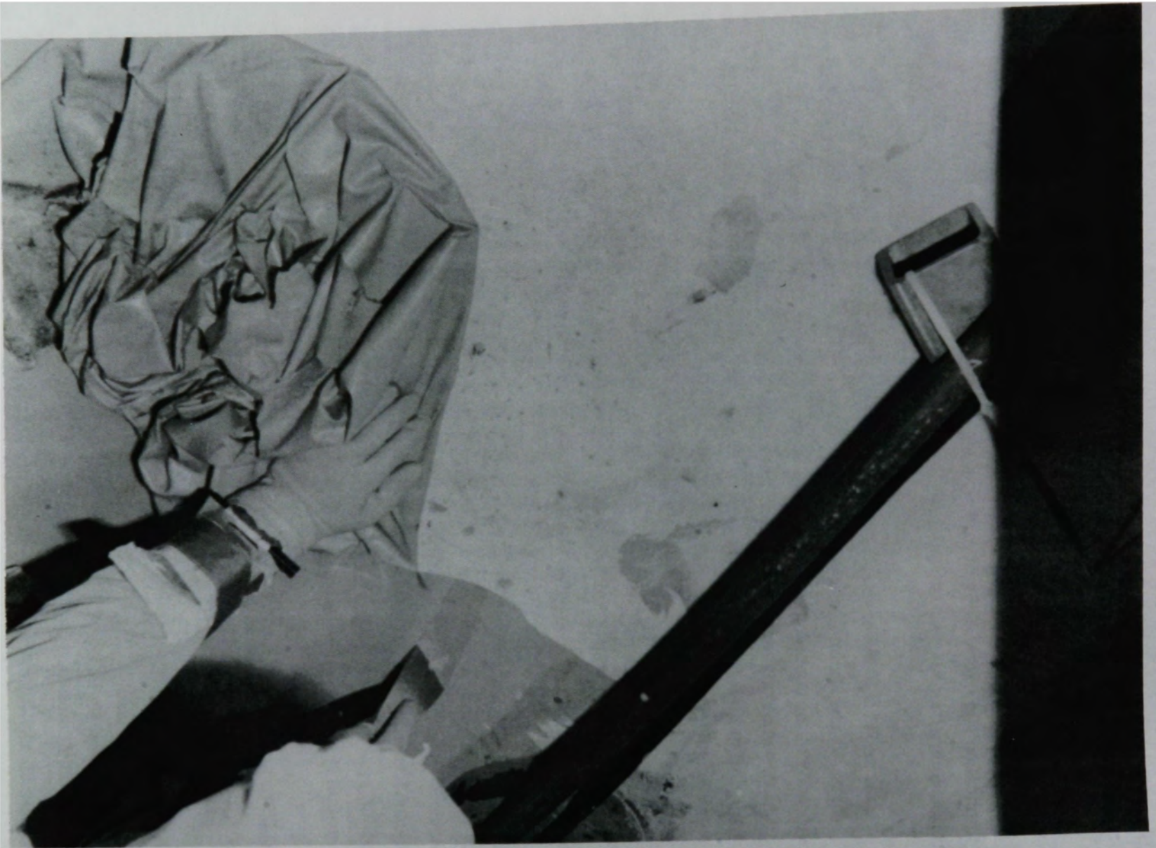
Figure 4. TMI-2 worker removing strippable coating from concrete floor.
